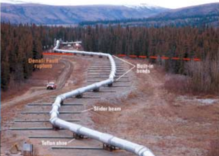
Fig. 3. View of part of the Trans-Alaska Pipeline at the Denali Fault showing major design features. Fault movement and intense ground shaking were accommodated by zigzagging the pipeline and leaving it free to slide by supporting it on Teflon shoes mounted on long horizontal steel slider beams that parallel the fault trend. This slider design was used in a corridor 1900 ft. wide to accommodate uncertainties in the exact position of the fault trace at the pipeline crossing.
